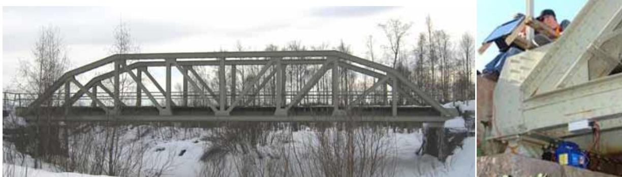
Figure 91 Event-based strain monitoring on a railway bridge with a PV panel [103]
